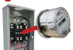
Insert meter back into meter socket with the Disconnect Sleeves in place.
