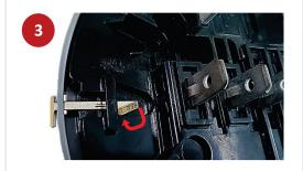
To lock seal, carefully lift tab (Fig. A) at the base of the seal to bend the base completely over (Fig. B) then fold the seal flag unto side of meter cover (Fig. C).
