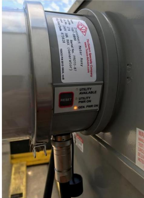
Picture 2: Gen/Battery Power ON
