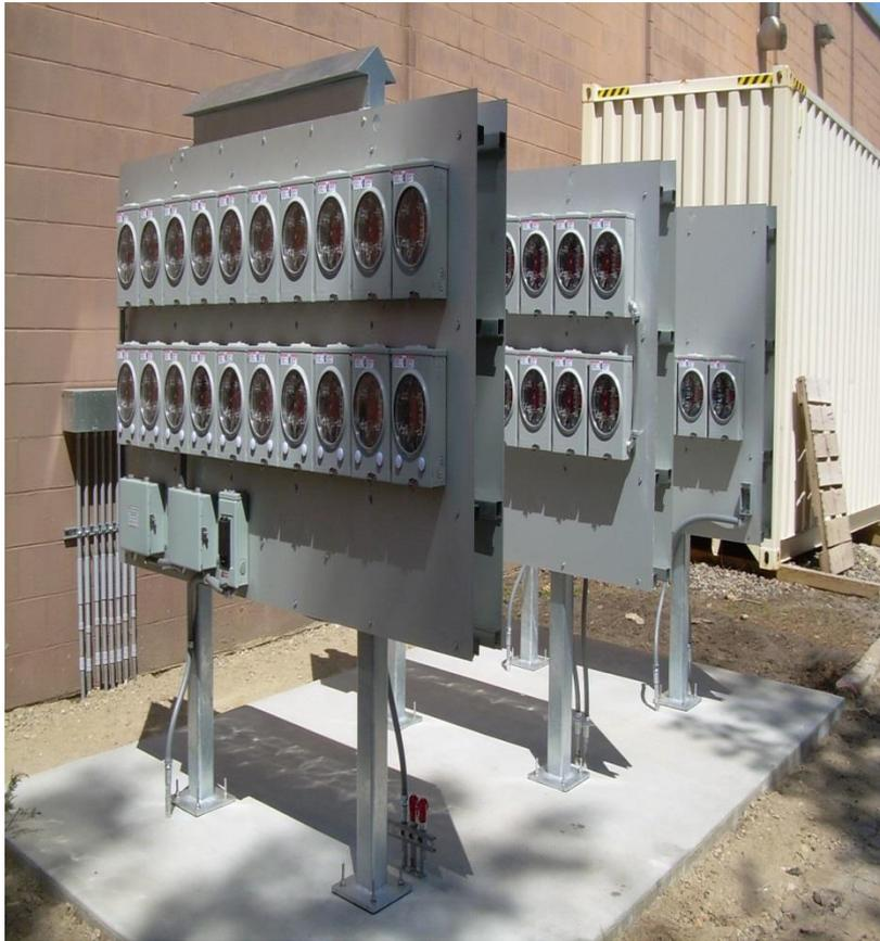
The meter farm gives you a microcosm of your population and as a result can be used as a baseline to ensure the longer term stability of the meters being delivered and to ensure that they are not changing over the course of the deployment.
