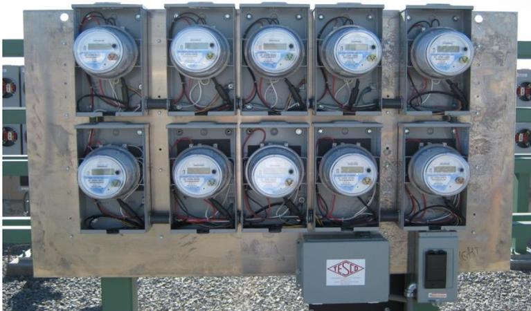
Prior to deployment you are still in Meter Certification mode. Much of this work is done on meter qualification boards, programming stations and meter test boards.
