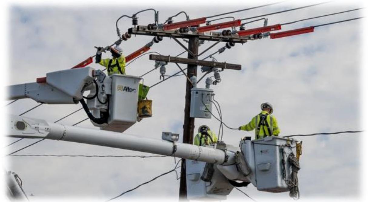
Utilities looking to modernize without replacing legacy systems
