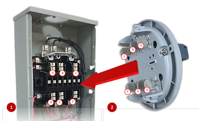
Locate and prepare meter socket where the meter socket jumper cover is to be inserted.
