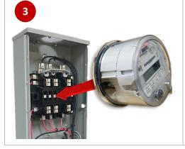
Insert meter back into meter socket with the Disconnect Sleeves in place.
