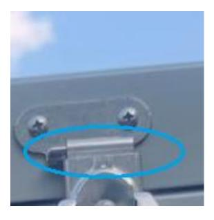
Spin the latches clockwise until the latch is aligned with the hole in the lock and place the latches down until they connect.
